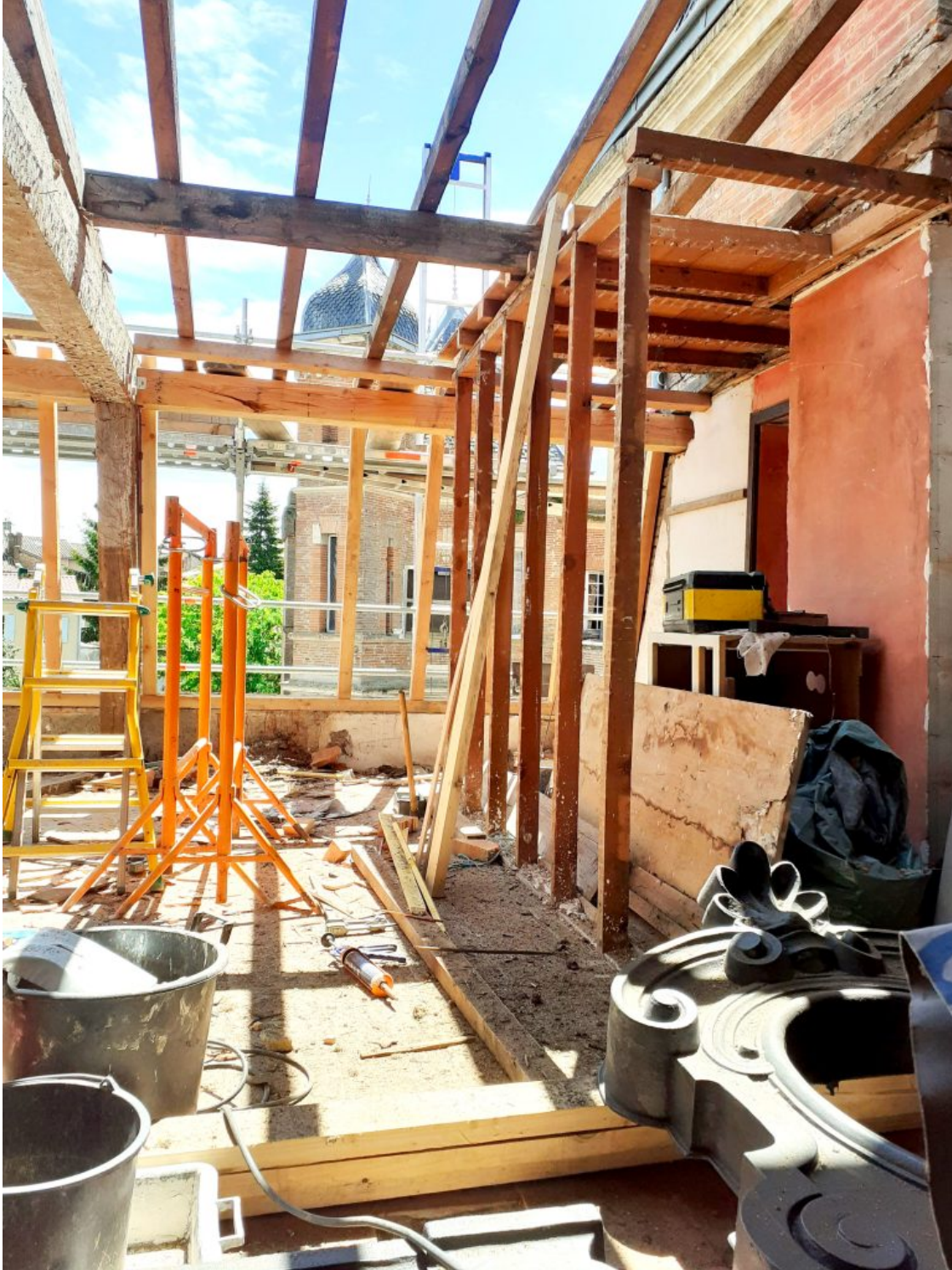
Chantier, 2021 © Alter Habitat Lislois
